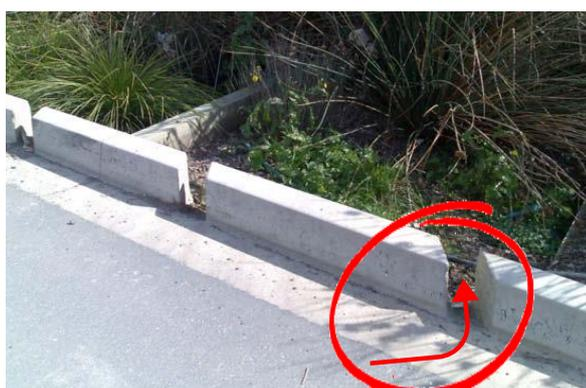
Incorporating on-site landscaping with stormwater management. This example captures runoff from parking areas, channelling it to a rain garden via kerb cuts to filters before discharging to the piped system.
